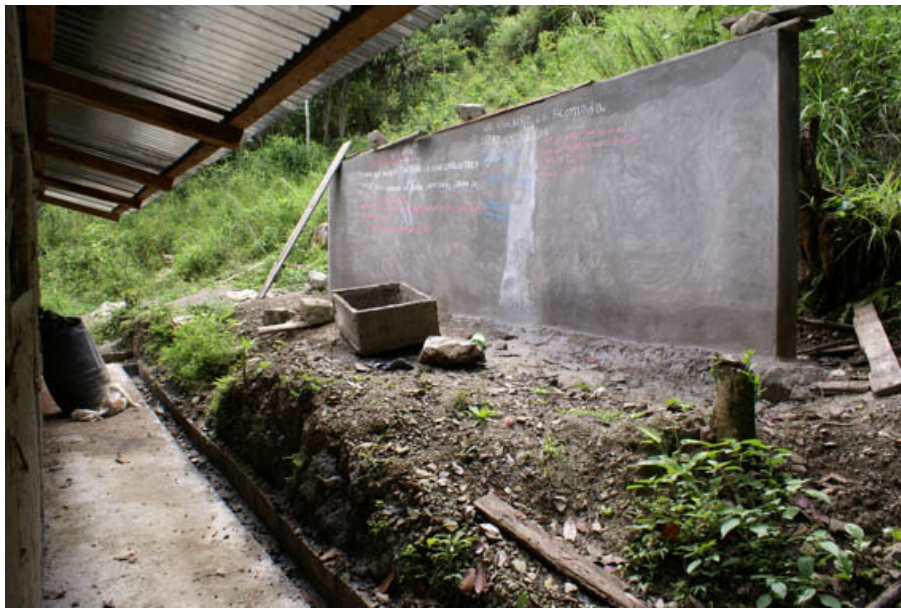
The new anti land slide retaining wall commissioned by the Foundations
