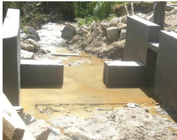
(Photos: Excavation of the conveyance ditch and the intake weir under construction)
